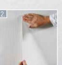
Hang the fabric length on the wall. During hanging, the fabric can be easily moved around and its position can be realigned.
