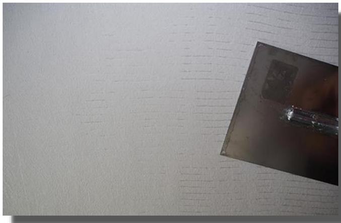
5.) A further levelling coat can be applied, depending on the surface requirements. Then sand off any remaining surface unevenness. Leave to dry fully before applying any further finish in accordance with the manufacturer's instructions.
