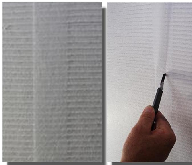
4.) Then smooth all over until the grooves in the levelling compound are no longer visible.
